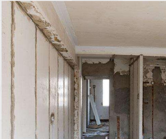
Old room transformation/ New toilet/Balcony/Garage
